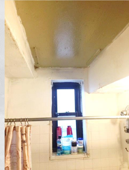
Full View: Bathroom Wall
