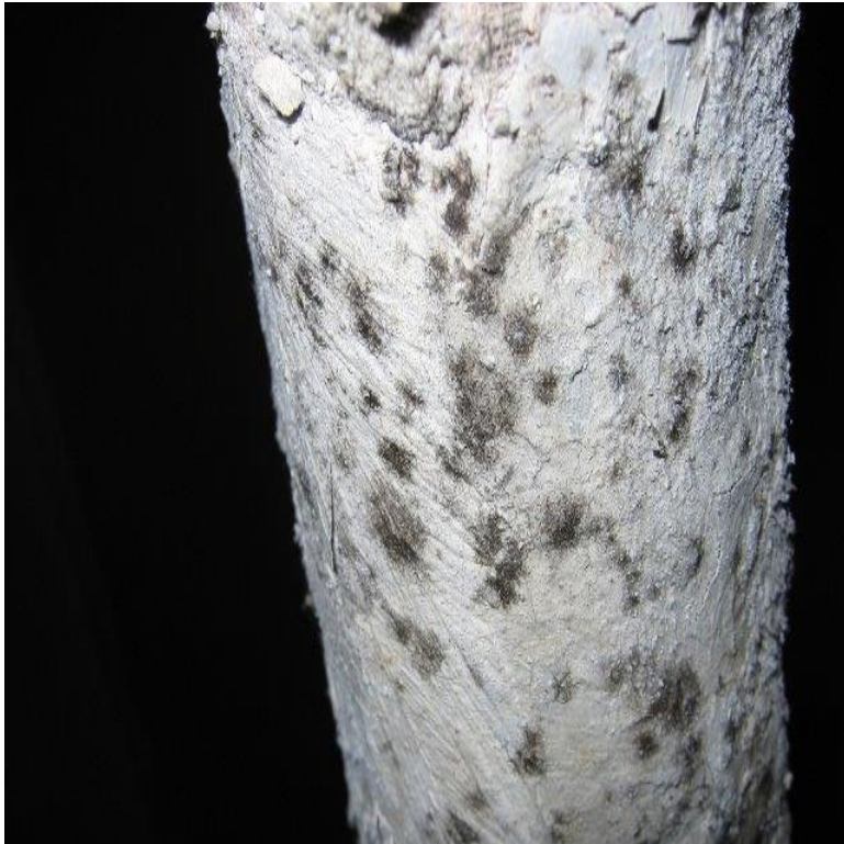
ACM- Pipe insulation (T.S.I)
