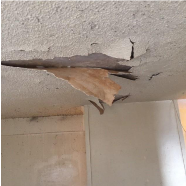
Close Up: Living Room Ceiling
