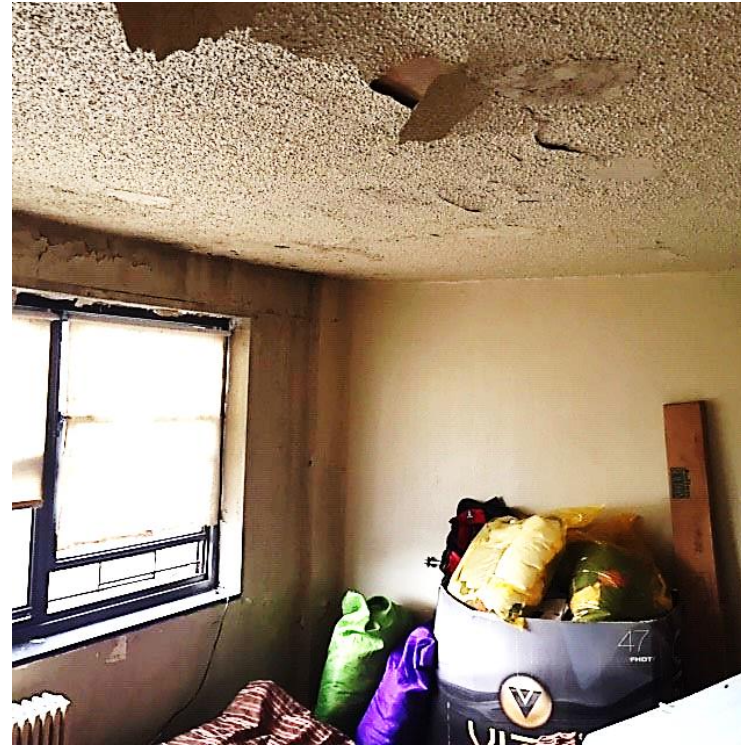
Full View: Living Room Ceiling
