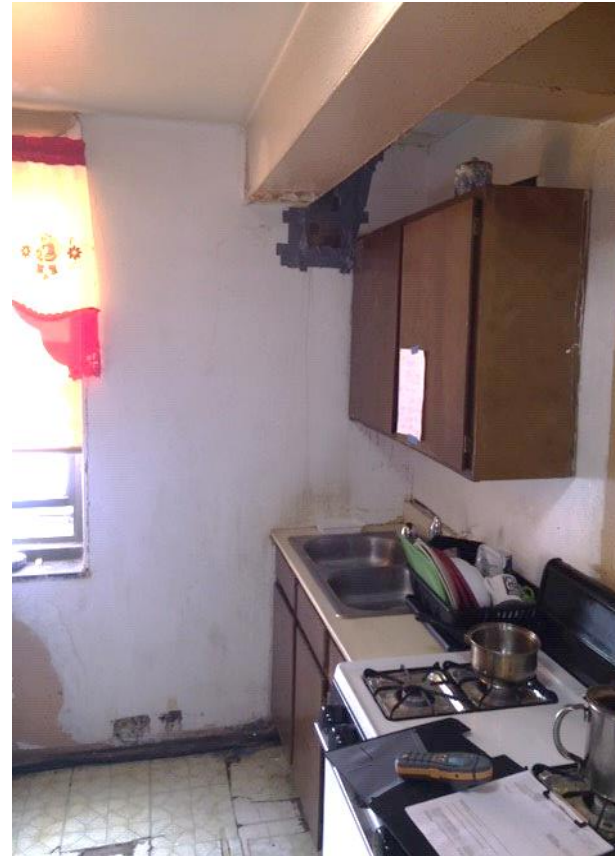
Full View: Kitchen
