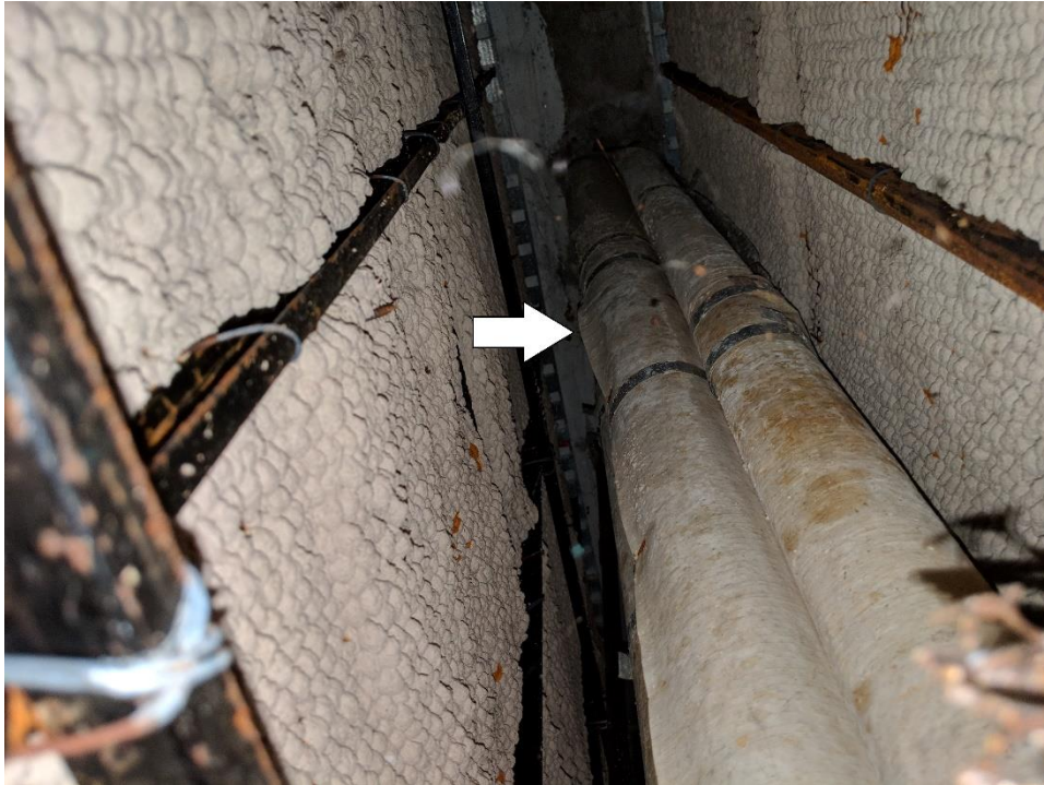
ACM- Pipe insulation (T.S.I)
