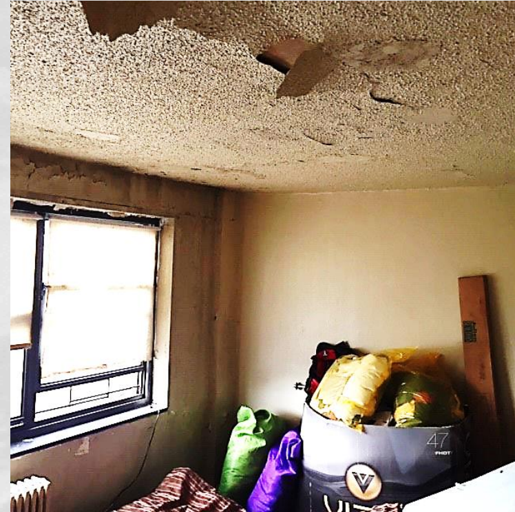
Full View: Living Room Ceiling
