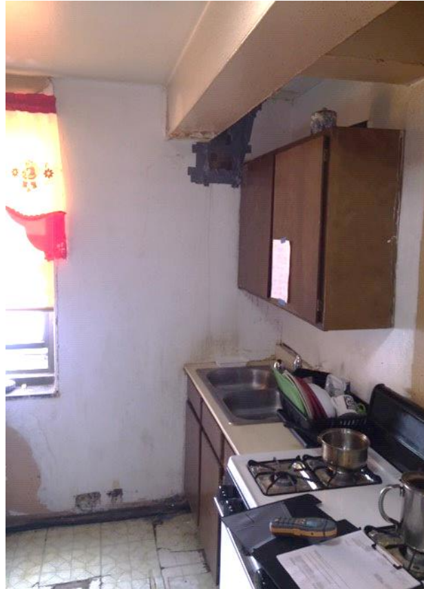
Full View: Kitchen
