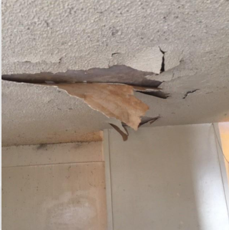
Close Up: Living Room Ceiling
