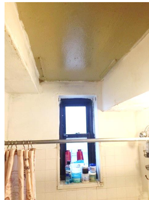
Full View: Bathroom Wall
